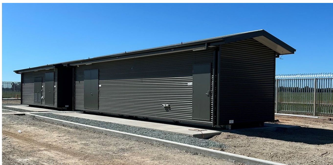
Plate 3 Example style of prefabricated building used at the nearby Quorn Park Switching Station
